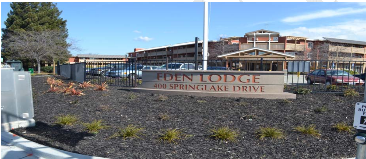
New, large vehicular entrances and gates
